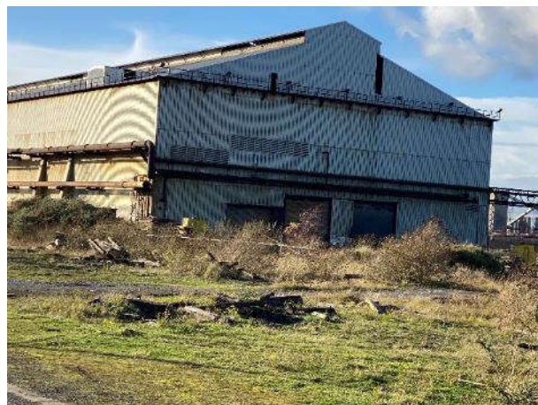
East Elevation of the Workshop
