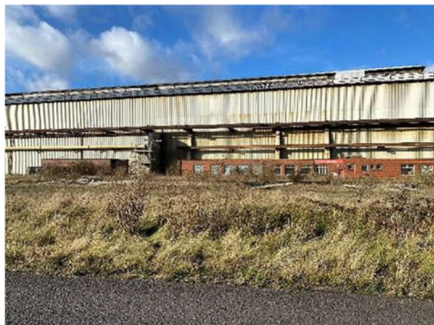
Offices and South Elevation
