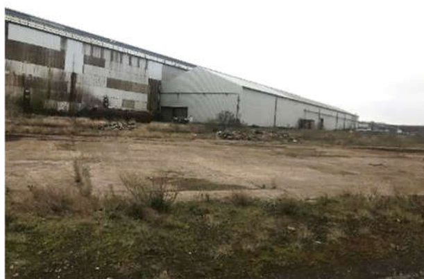
Boiler House Structure
