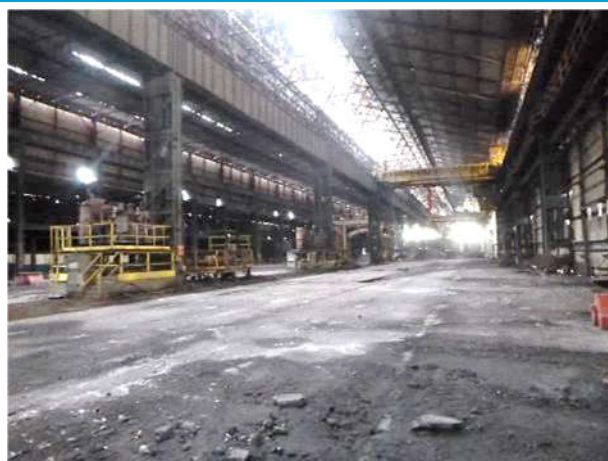
Internal view of Overhead Crane.
