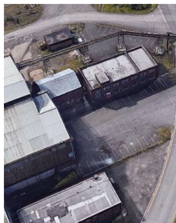
Office and Amenity Block view to the south.
